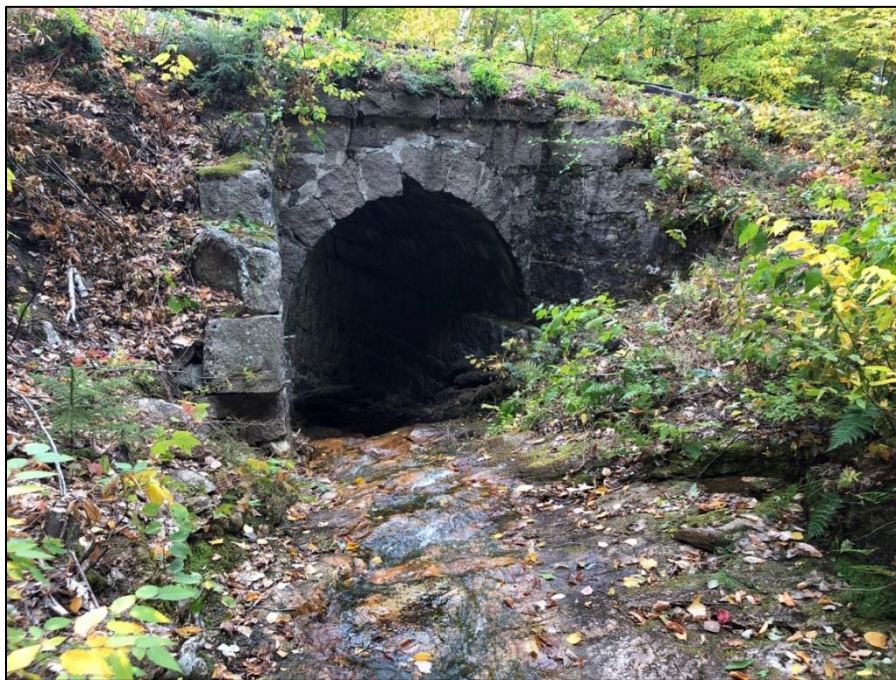
Figure 8: Kedron Brook Railroad crossing.
