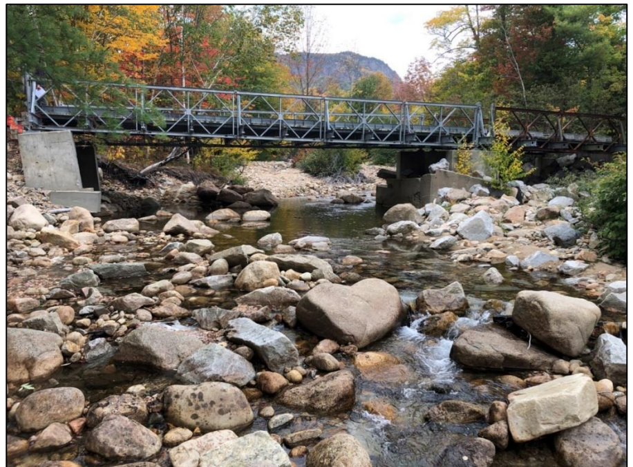
Figure 7: Failing Bridge over Bemis Brook providing access to private property.
