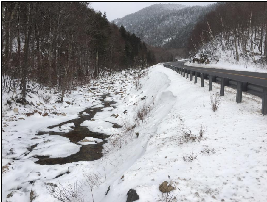
Figure 4: Location of little buffer between on US Route 302 and the Saco River, Hart's Location during winter conditions.
