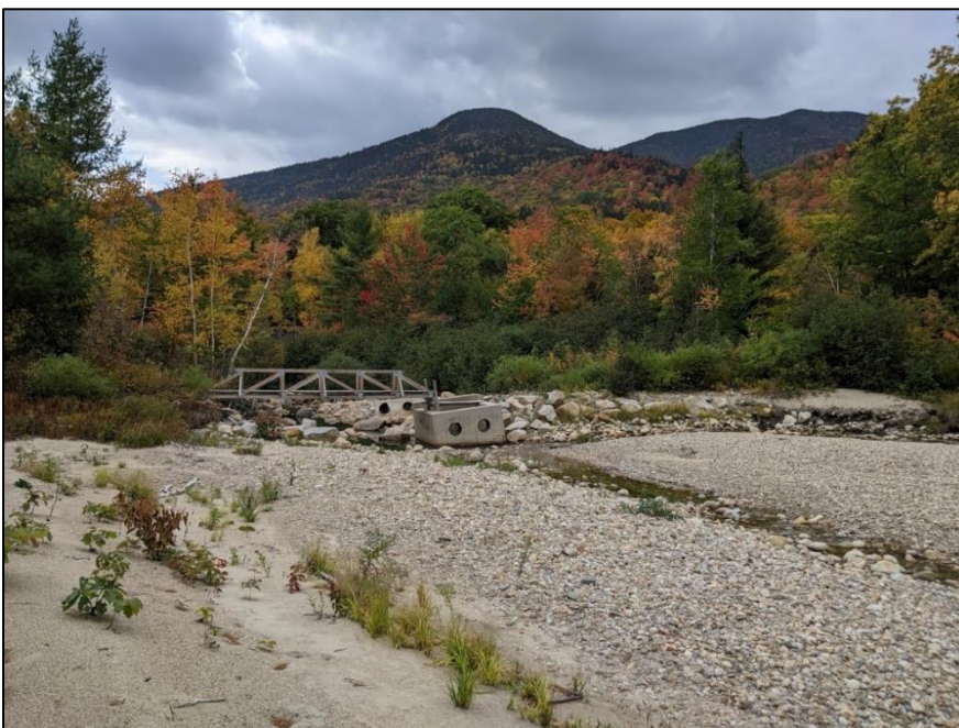
Figure 5: Secondary channel of the Saco River at the private property situated between Bemis Brook and the Saco main channel. The dam previously impounded streamwater into a reflection pond, but was destroyed by flooding in Tropical Storm Irene.
