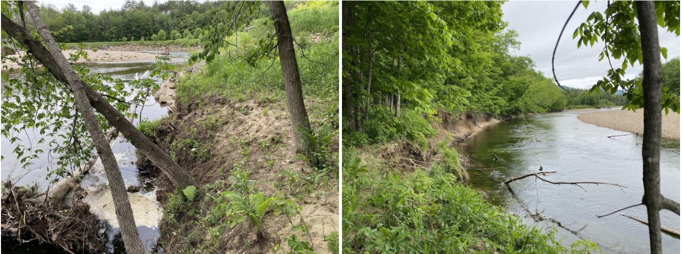
Left: Photo of a hard armored bank with erosion directly above it, likely a result of the Saco's erosive power being directed upstream. Right: The eroded banks continue approximately 800 feet upstream (Credit: FBE).
